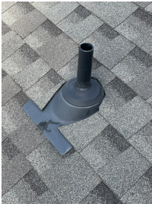
Missing diverter flashing
