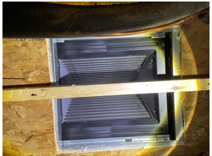
Evaporator coils
