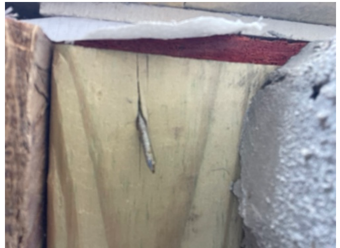
Exposed sill plate
