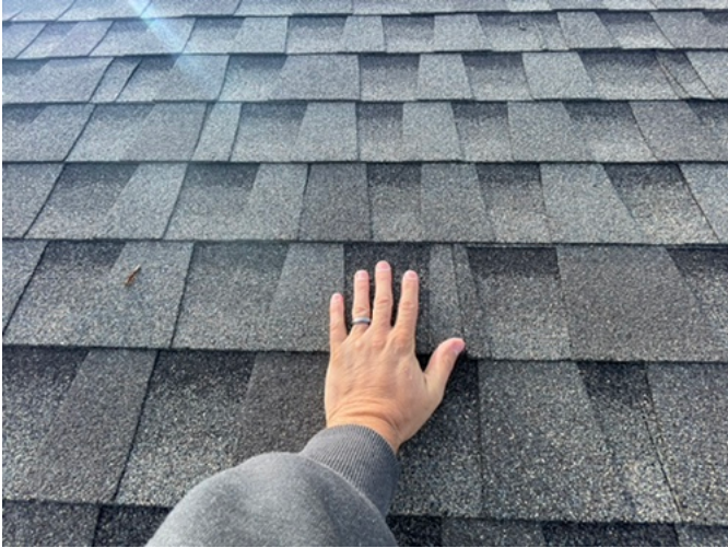
Asphalt dimensional shingles
