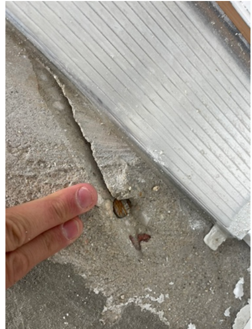
Cut J bolts for wall attachment
