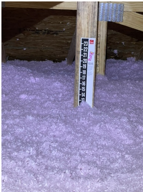
13" of loose insulation
