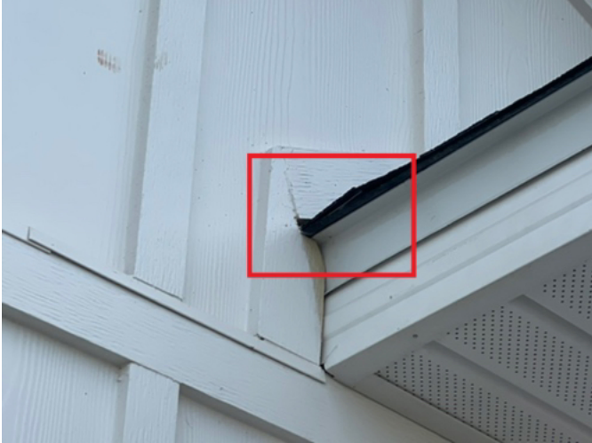
Missing diverter flashing
